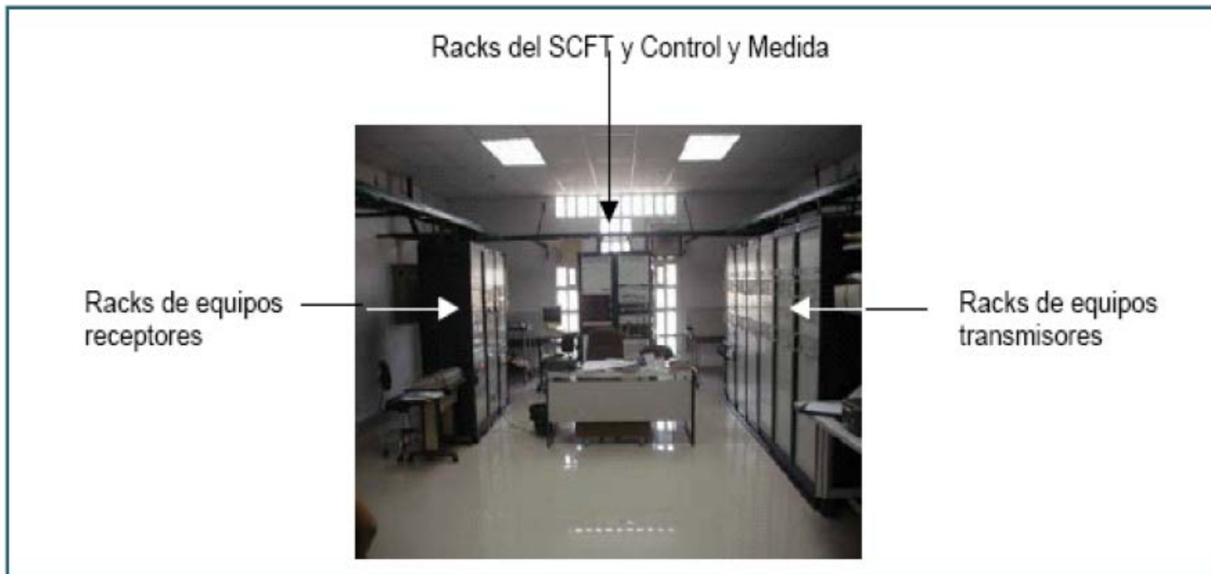
Cáceres communication centre
